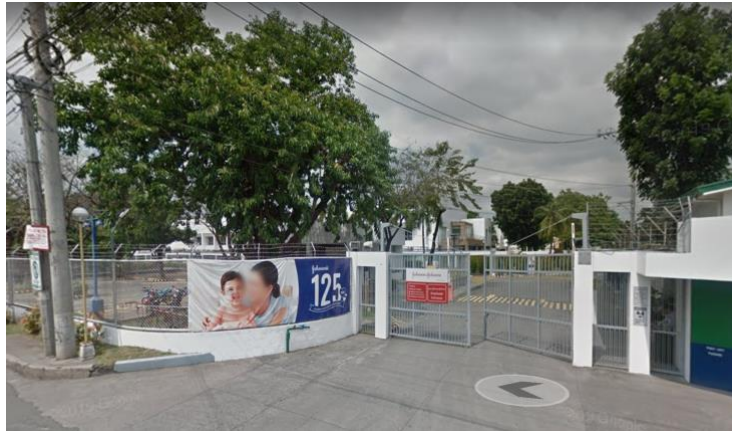
Entrance of J&J baby powder plant, Parañaque City, Philippines. Google Maps Streetview.
